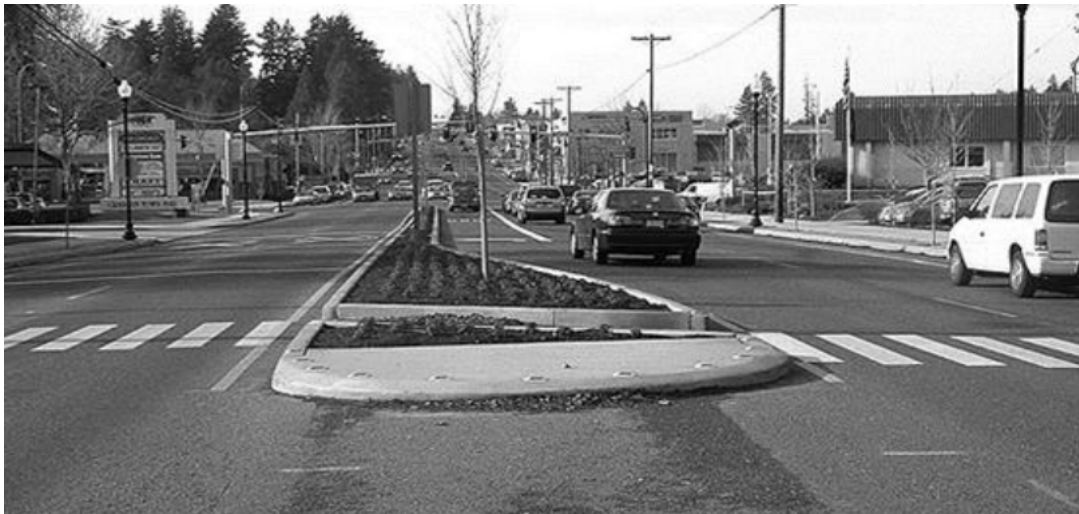
Figure 2. Median nose extended beyond the crosswalk to provide an enclosed pedestrian refuge. Source: Kimley-Horn and Associates, Inc.
