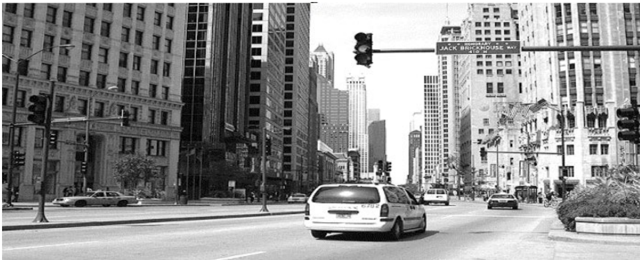
Figure 1. Narrow medians, such as on this boulevard in Chicago, should only be used to restrict turning movements, separate opposing traffic and create space for traffic control devices. Source: The Congress for the New Urbanism.
