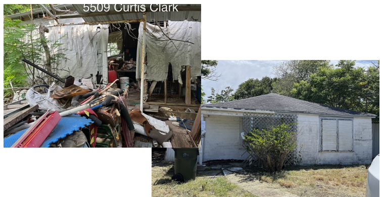
Curtis Clark before & after abatement
