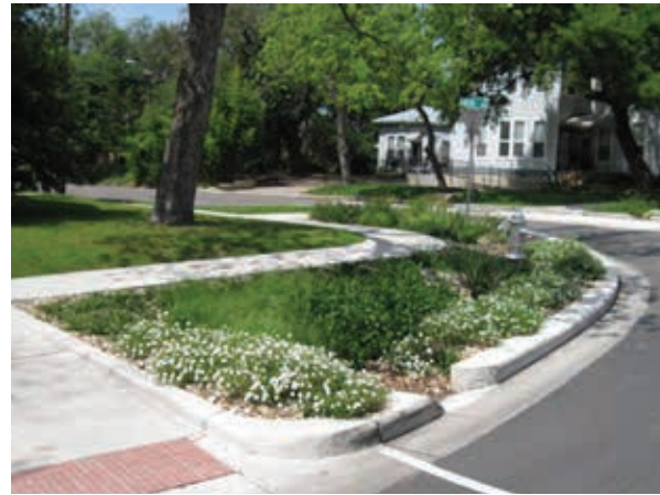
Example of Bioswale
