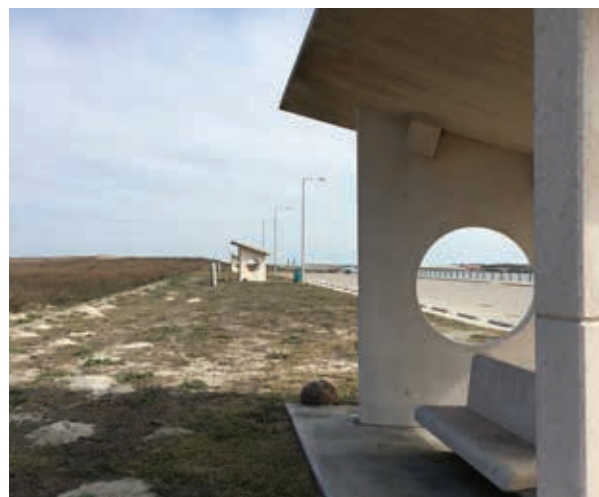
Packery Channel Recreational Facilities
