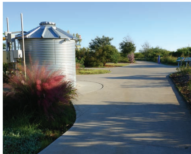
Oso Wetlands Preserve Rainwater Cistern
