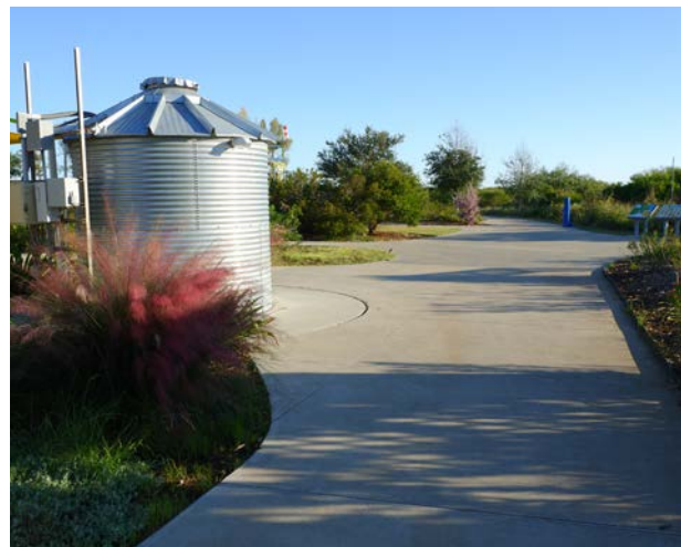
Oso Wetlands Preserve Rainwater Cistern
